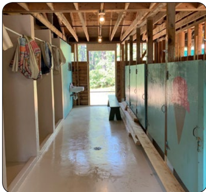
Bath house renovations include more screens; new exit doors; new flooring for cleaner, drier floors; and making wood surfaces easier to clean by polyurethaning them.
