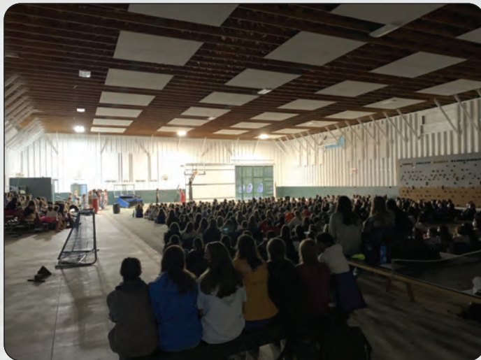
Acoustic panels on the ceiling of the sports complex have greatly improved all-camp gatherings.
